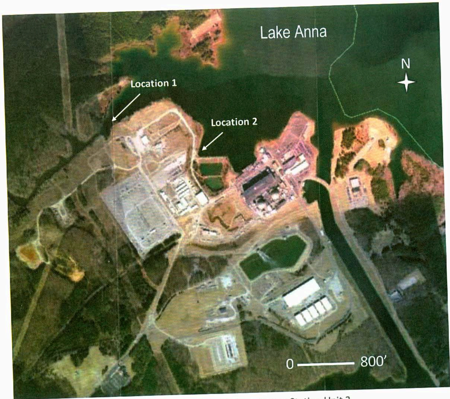
Figure 1. Proposed North Anna Power Station Unit 3 Potential Water Withdrawal Locations for Construction Activities
